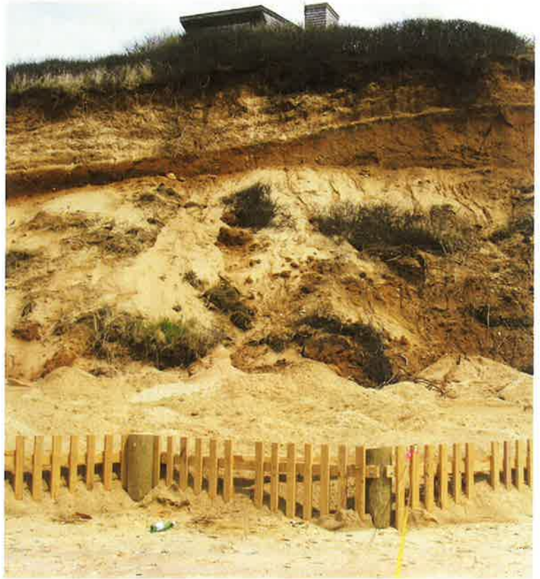
Eroding coastal bank pre-coir envelopes (2011)
